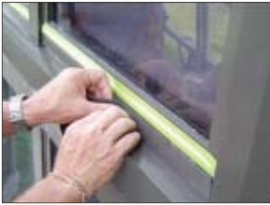
Pre-cured silicone sealant installed in an aluminum window system
