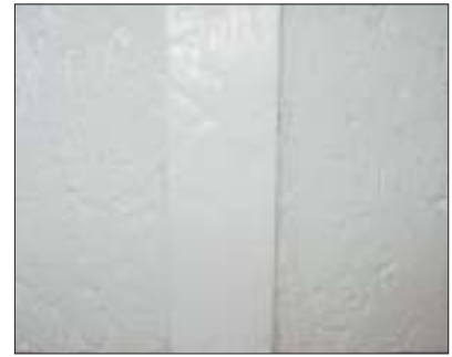
EIFS joint repaired using textured pre-cured silicone sealant
