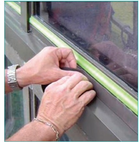
Pre-cured silicone sealant installed in an aluminum window system.
