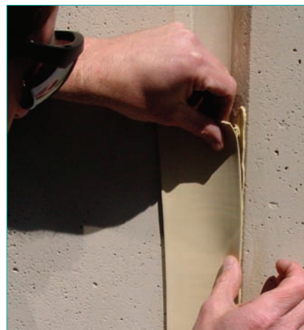
Repair joint installation
